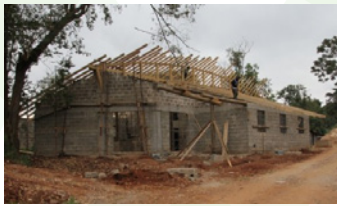
Construction de la nursery
